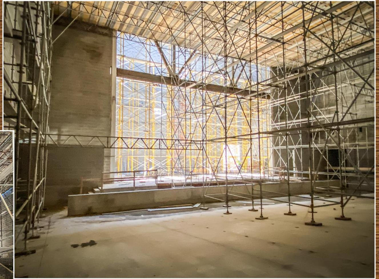
**Scaffolding in the PAC interior and fly loft is being prepared to begin work on the above ceiling.**
