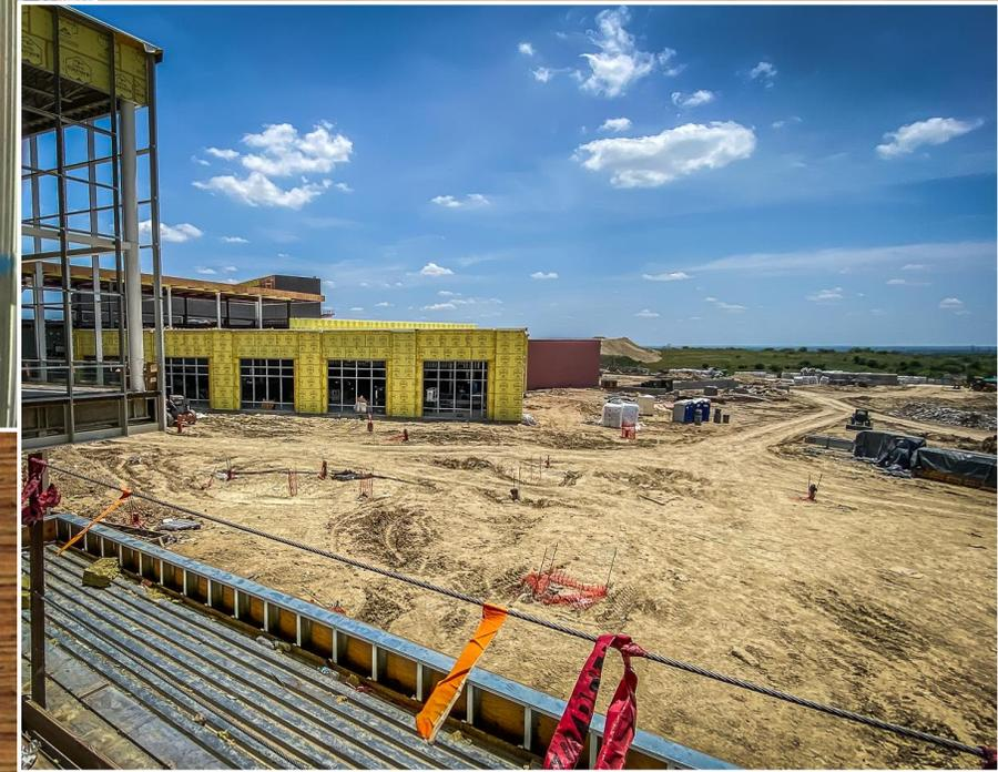
**Academic areas are progressing in different stages in the 100, 200, and 300 hallways, which includes: framing, utilities, sheetrock, tape and bedding, blocking for monitors, duct work, and electrical work.**
