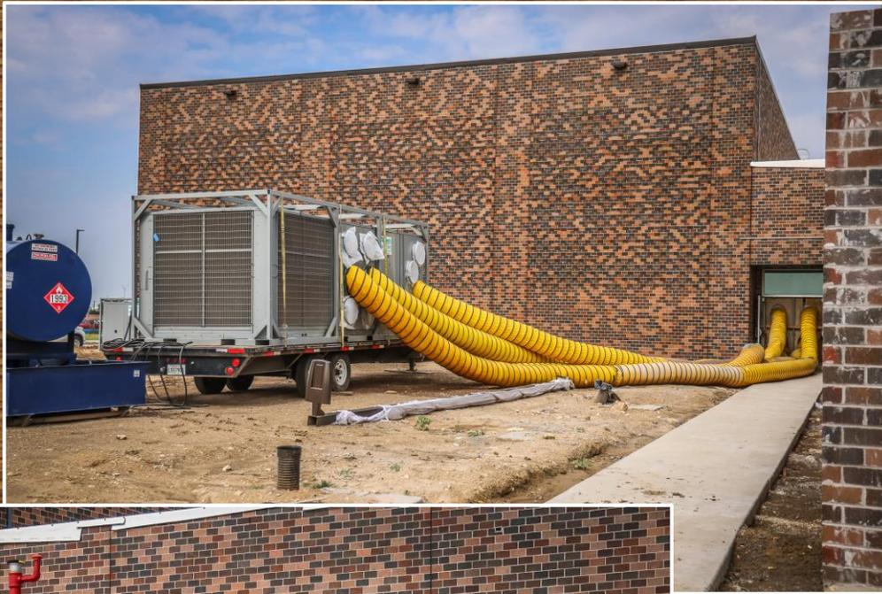
Light pole installation has started in the landscaped area in the front of the campus. The fire pump was set in the delivery yard on the east side of the building. Temporary HVAC has been set up to climatize area A and B for flooring installation.
