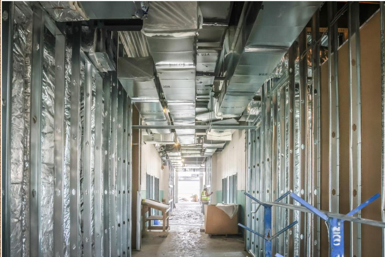
**Duct work and sheetrock installation continue in area D2.**
